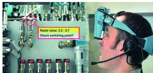
Figure 2.2: Augmented reality helps Fabio troubleshoot the installation
